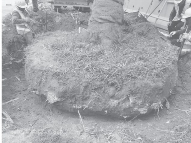
Fig. 1.8 Root ball excavation
