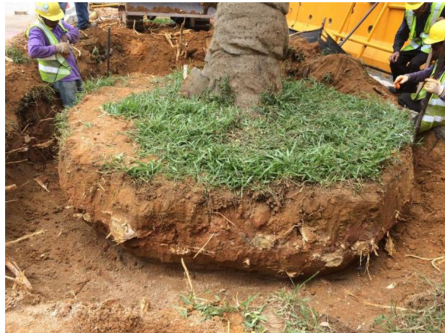
Fig. 1.8 Example – Root ball excavation
