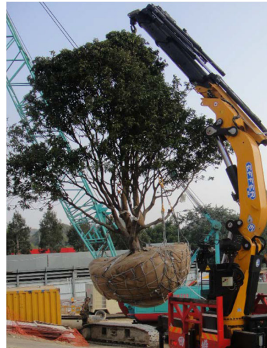
Fig. 1.9 Example – Root Ball excavation and Burlap, and lifting and moving
