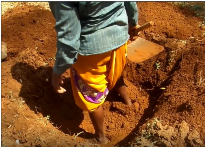
Fig. 1.6 Preparation of pit
